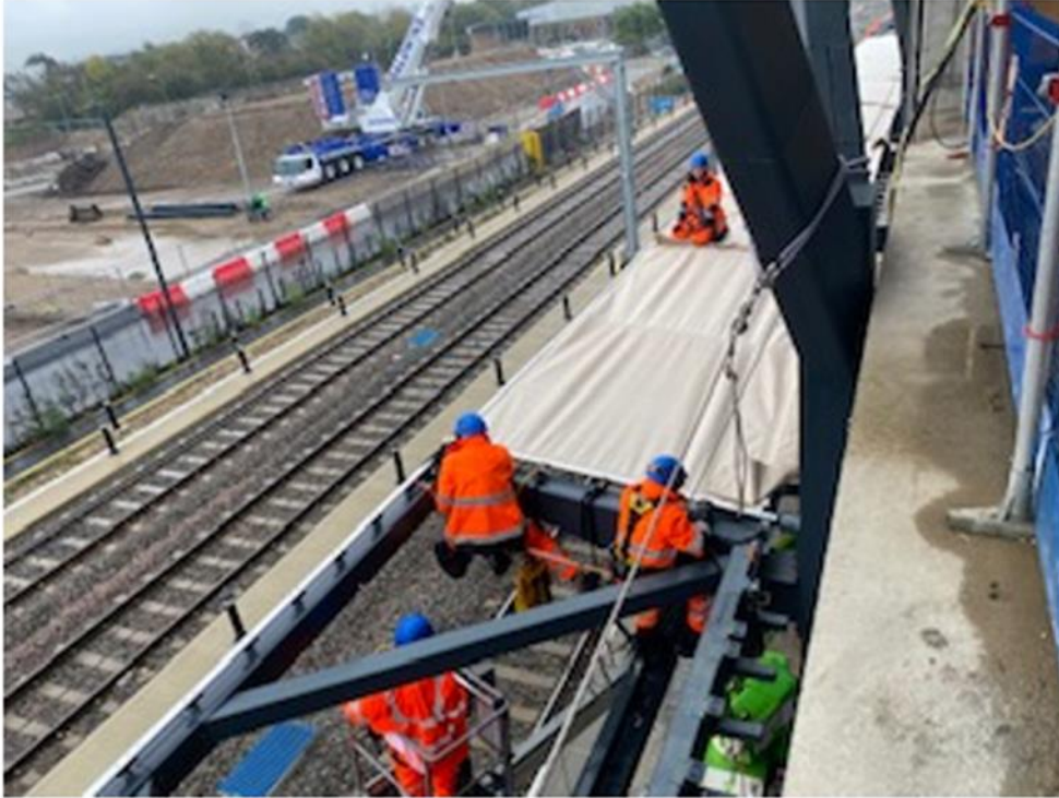
Canopy roof sheeting in possession to lower platform canopies 30% complete.
