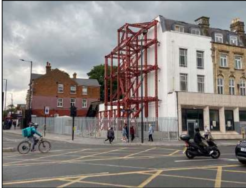
Figure 2: Current propping system at site
